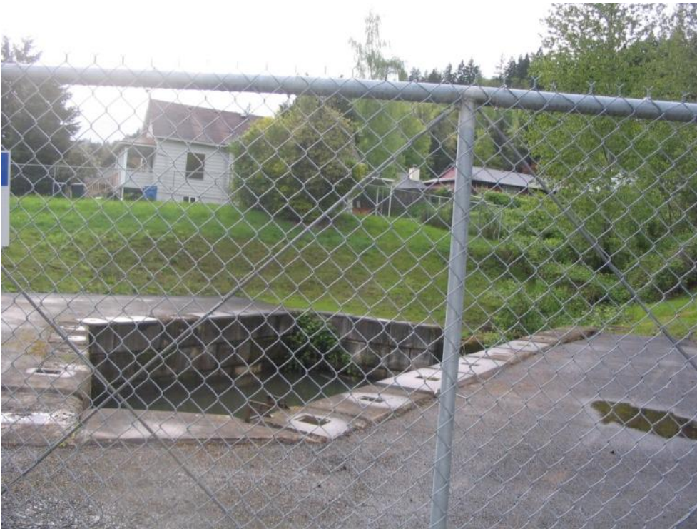
Figure 5-4: Sediment collection facility at Blue Creek.
