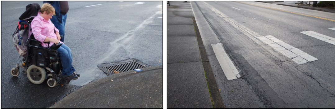
Figure 6: Examples of levels of accessibility experienced during the CAC field tour, such as a missing ramp and a ramp with an outdated design
