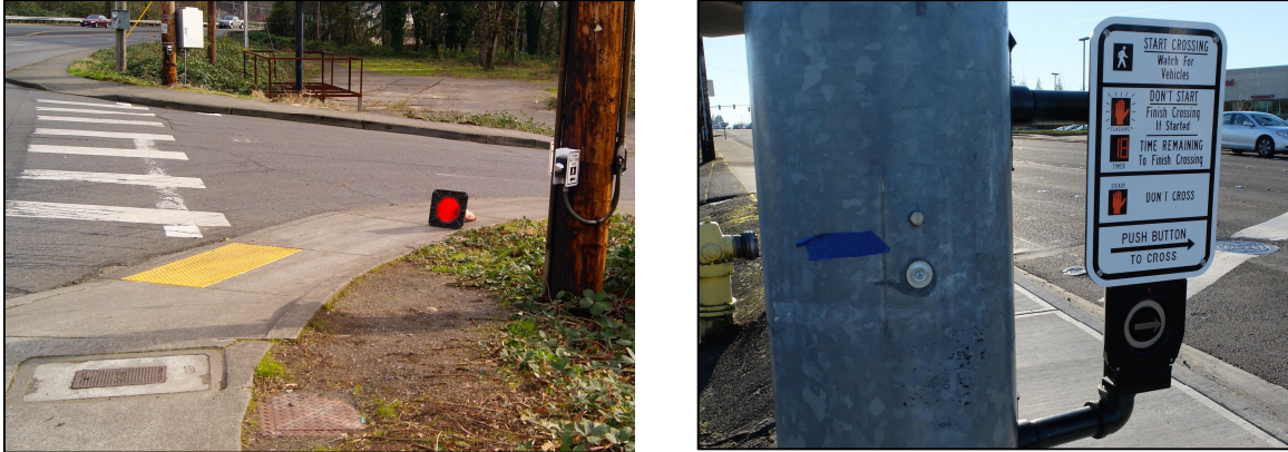
Figure 3: Examples of pedestrian push buttons, inaccessible versus accessible
