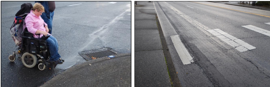
Figure 6: Examples of levels of accessibility experienced during the CAC field tour, such as a missing ramp and a ramp with an outdated design
