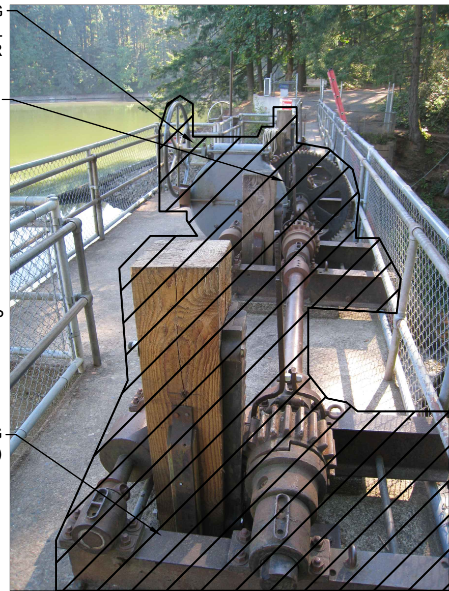
EXISTING UPPER DAM SPILLWAY GATE HOISTS
