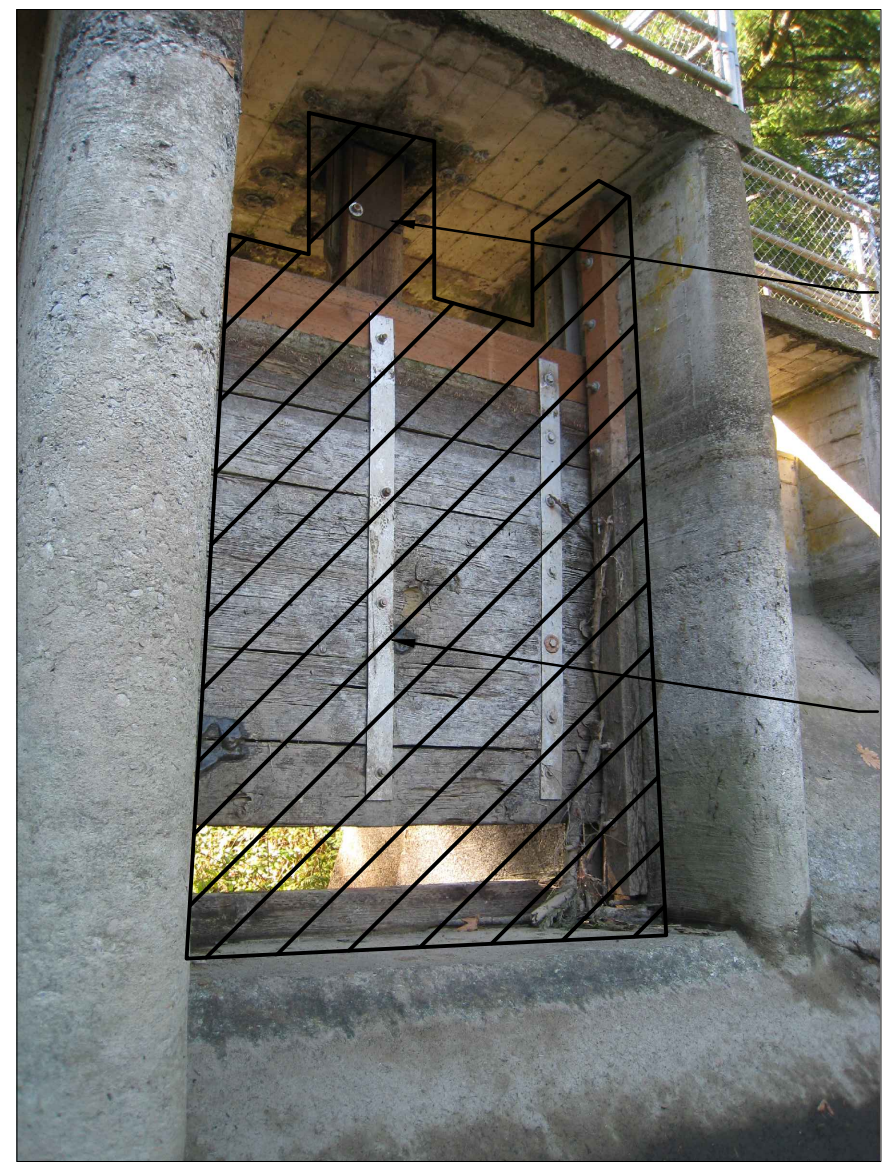
EXISTING UPPER DAM SPILLWAY GATES (UPSTREAM SIDE)
