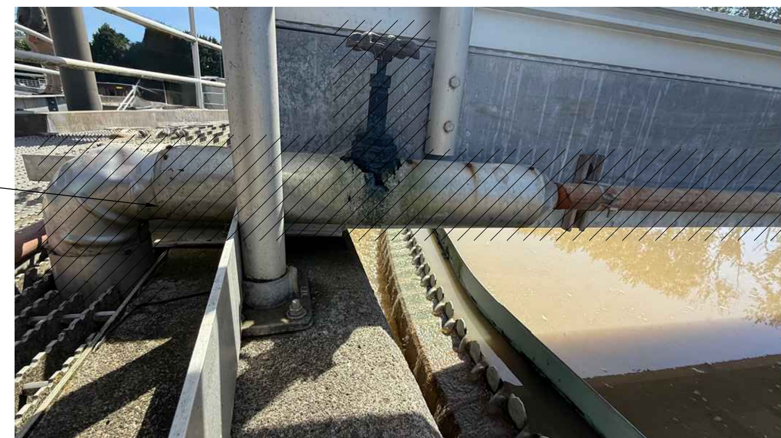
CLARIFIER SPRAY BAR DETAIL
