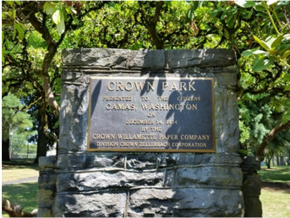
Photo 3. Basalt entrance monument in the southwest corner of Crown Park. The view is towards the northeast.
