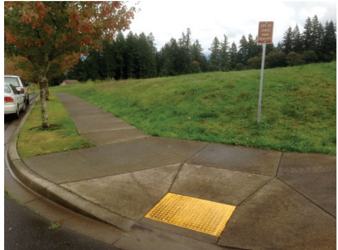
Pedestrian access at NW 27 th Avenue
