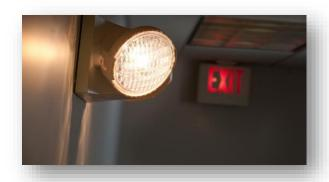
Egress lighting provides a clear view of the path of egress, enabling occupants to leave a building during normal circumstances when occupied.
