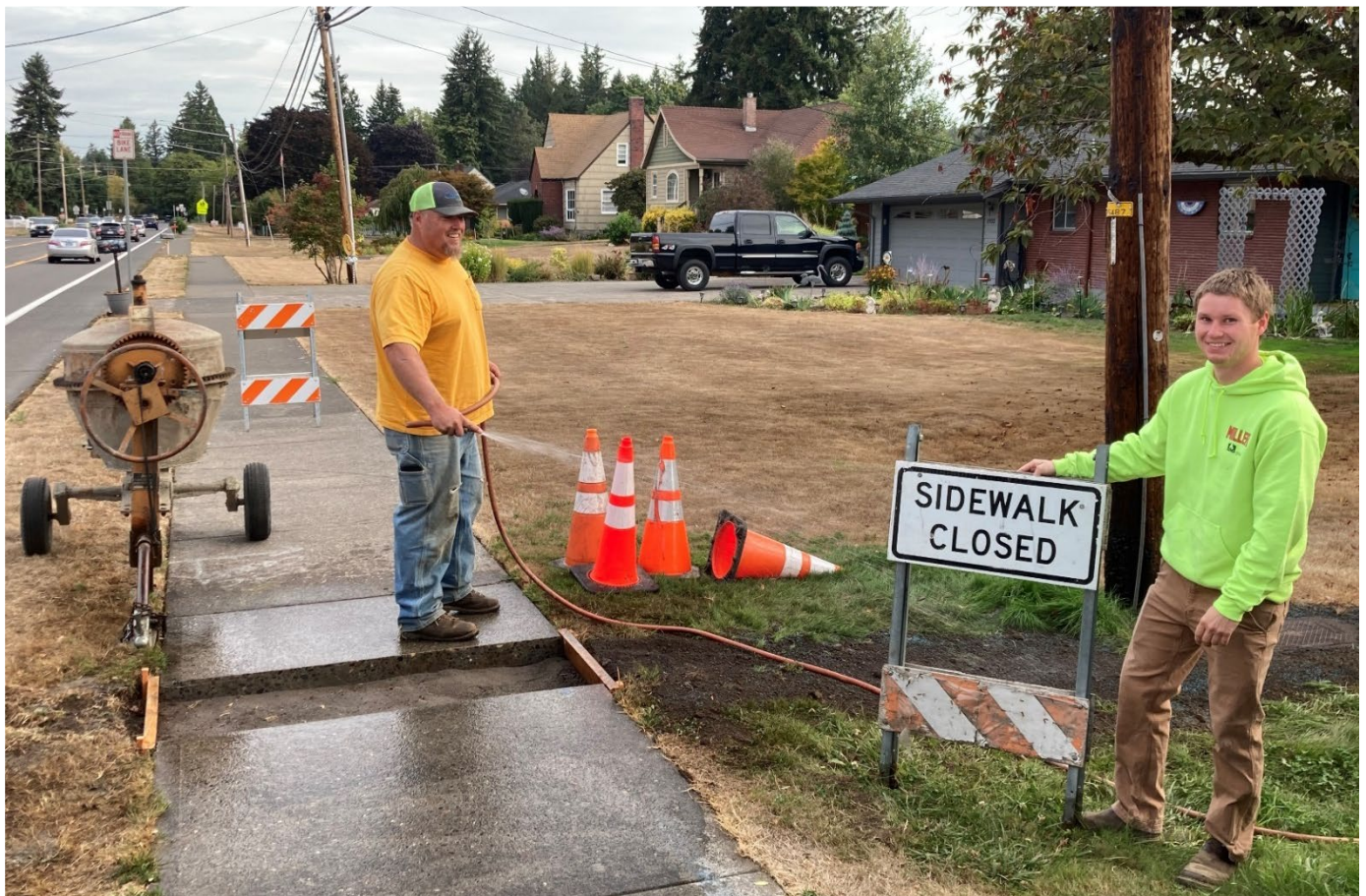
City staff repair the sidewalk following waterline maintenance
