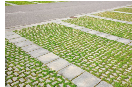
Driveways using permeable pavers (Source: © Francesco Scatena/ Adobe Stock)
